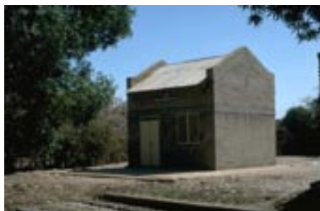
Figure 8.6 Well insulated tree seed store; the Sudan.
