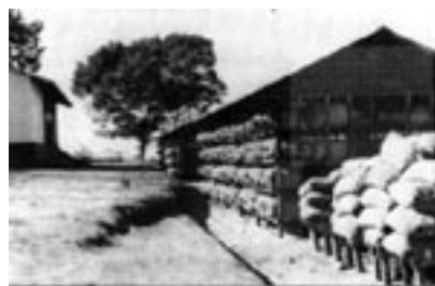
Figure 6.2. Pre-curing sheds with open-air racks; Zimbabwe
